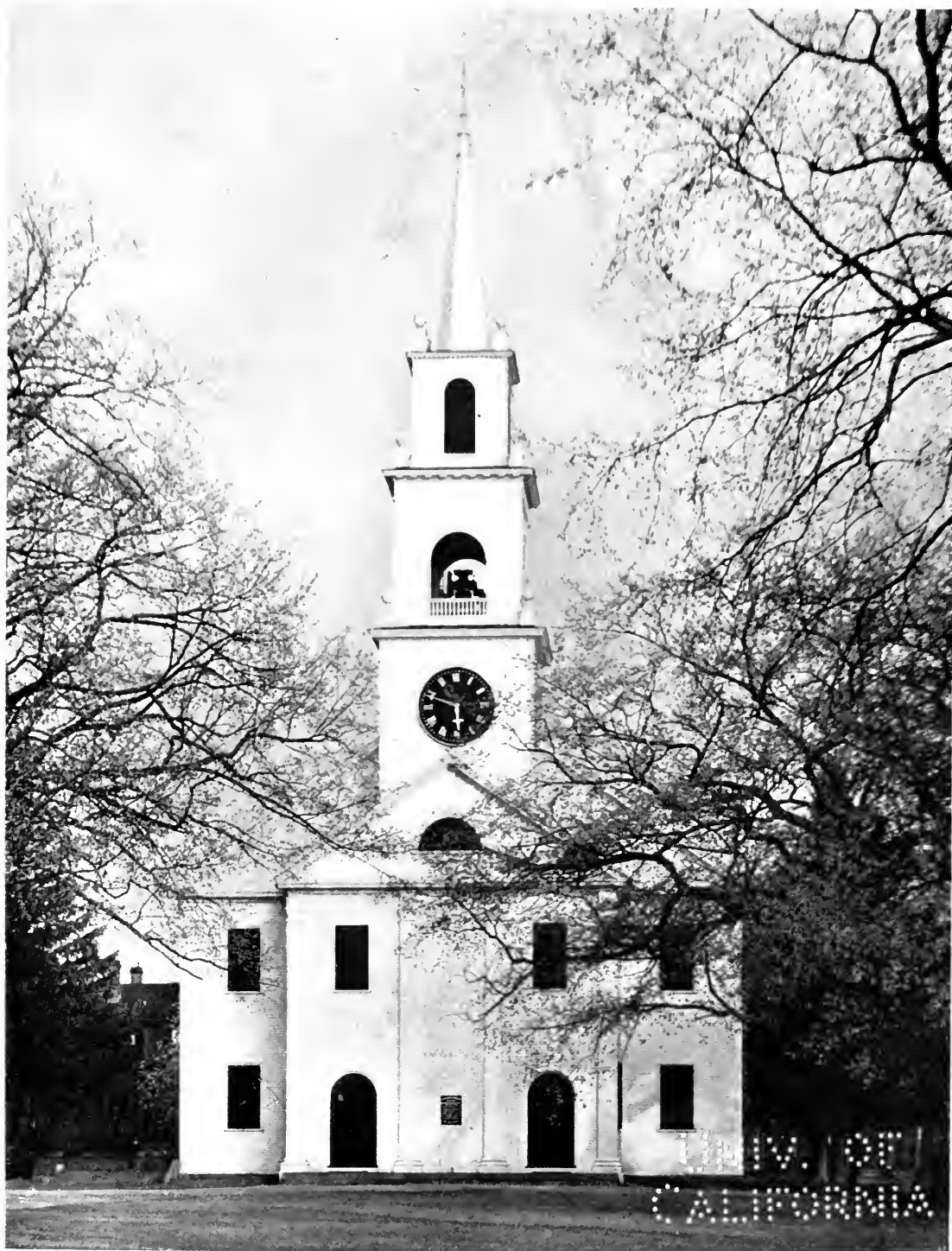
FIRST CHURCH, DEDHAM, MASSACHUSETTS Whose vestry is larger than the original meeting house of this society
